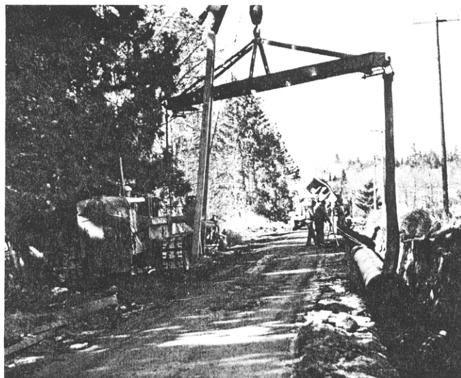
Pipe-laying cost is but one rural water-system factor.
