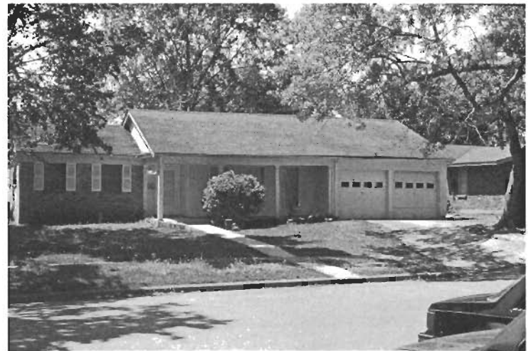
1984: House 5 years after foundation repair (photo by C. Norman)
