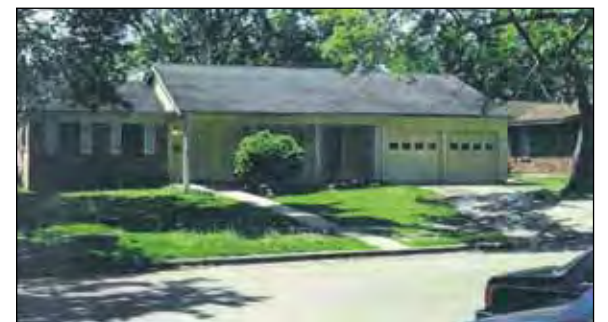
House five years after foundation repair (1985). Photo by C. Norman.
