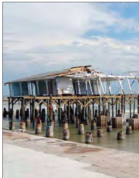
The Galveston sea wall does not help much if you are on the wrong side of it. This gift shop lost its windows and walls during Hurricane Ike. But at least it fared better than its neighbor, a restaurant, the only remains of which are the broken pilings in the foreground. Photo by Chris Barker.
