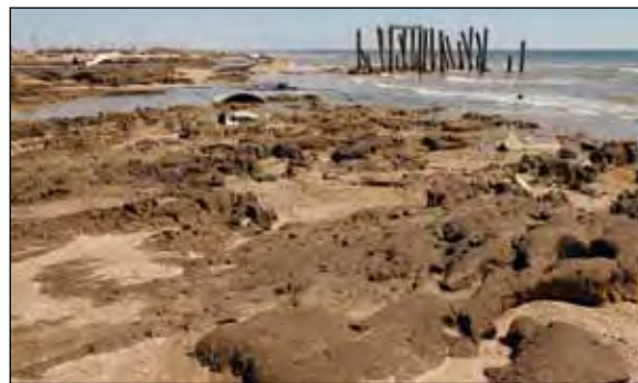
Destruction behind the Geotube after Hurricane Ike hit Gilchrist, Texas. The only structure on the beach that remained partially standing were the stilts of a beach cabin that was located seaward of the protective Geotube. Photo by Richard A. Ashmore.
