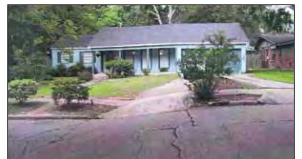
House with recurring foundation problems (2003). Photo by TSI.
