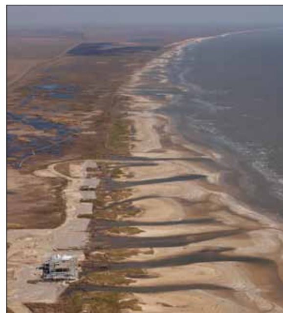
Sea Rim State Park, Texas, after Hurricane Ike. Photo by Richard A. Ashmore.
