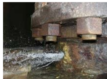
AP – This photo made available by the Nuclear Regulatory Commission shows a 10-gallon-per-minute leak which ...
