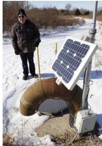
AP - In this Tuesday, Dec. 14, 2010 photo, retiree Bob Scamen stands near a discharge pipe for the Braidwood ...
