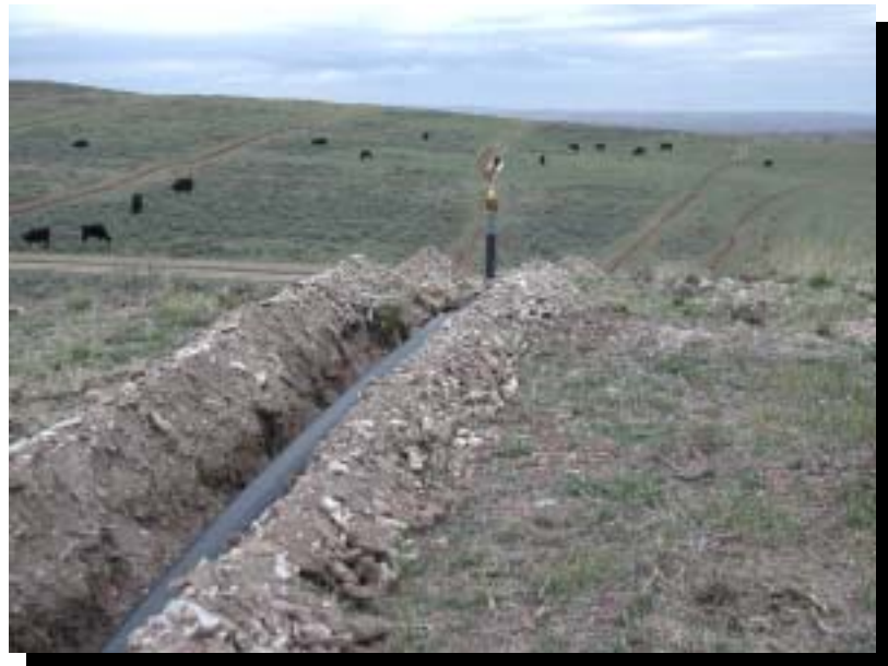
CBM water is piped to fields to be used for irrigation in this solid-set system. Note the use of “water cannons” attached to the PVC pipe. This method of irrigation has proved to be very cost-effective.
