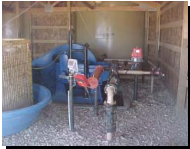
Injection well facility in the Powder River Basin
