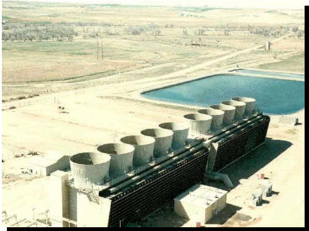
Power plant cooling tower.
