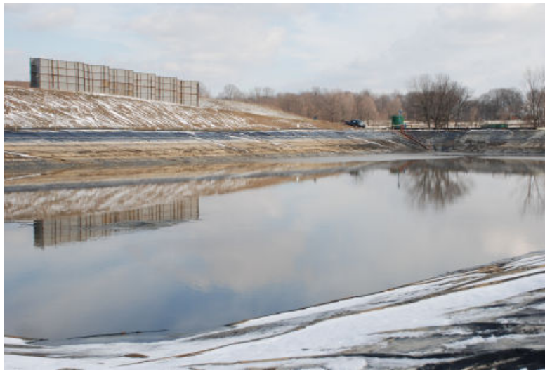
Figure 5.5: Evaporation pits are used to manage flowback water in Western states.
