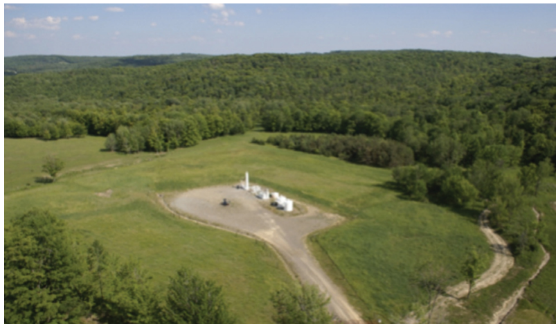
Shale gas well in production in the Marcellus area. The well head is seen in the middle of the pad. To the right is shown separation equipment and tanks for storing produced water before being further treated. (photo: Statoil/Chesapeake)
