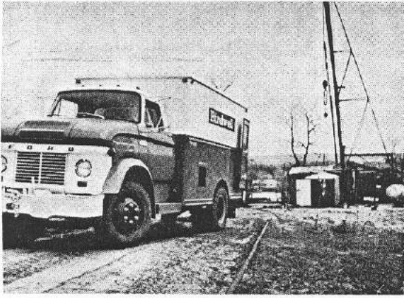
Logging truck in position to log hole. Cable-tool rig over drill-hole.
